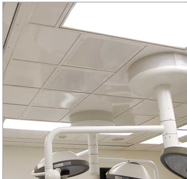
figure 1. This image illustrates the Linear Diffuser, Unitee CR Cleanroom System and Laminar Flow Diffusers.
