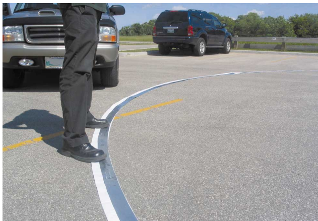
Custom Flow sheet steel templates were laid out at Price Winnipeg, which facilitated accurate visualization and measurement prior to manufacturing & installation.
