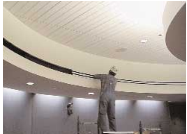
Custom Flow diffuser being installed.
