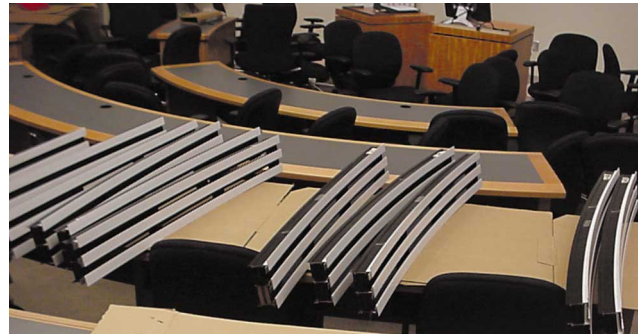
Some of the 208 Custom Flow segments that were needed to complete the ventilation in the lecture halls.
