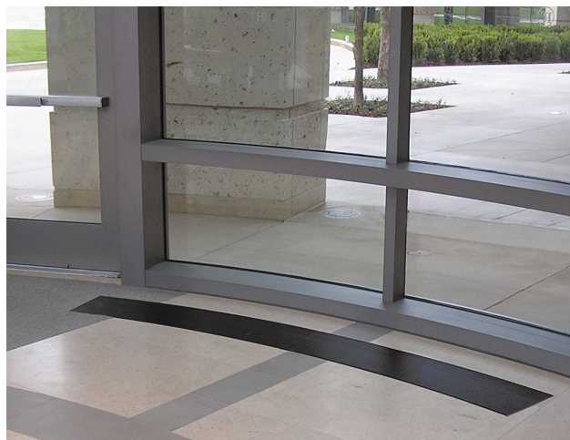
LBMH installed in the marble lobby floor
