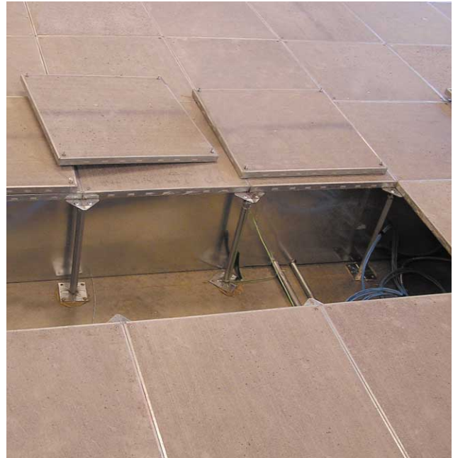
Underfloor System with Plenum during installation.
