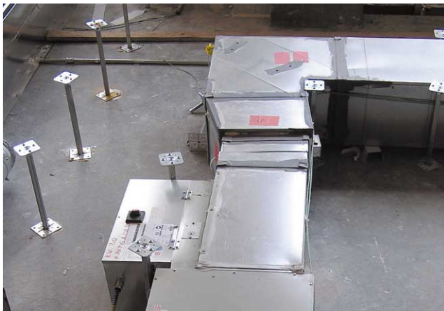
Underfloor System during installation.
