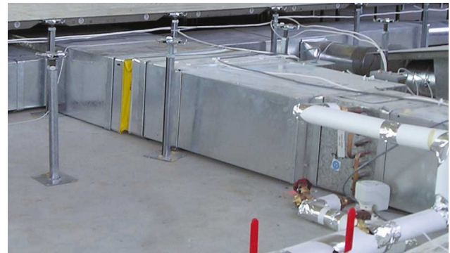
Head on view of the raised plenum holding the Underfloor System and Terminal Unit products.
