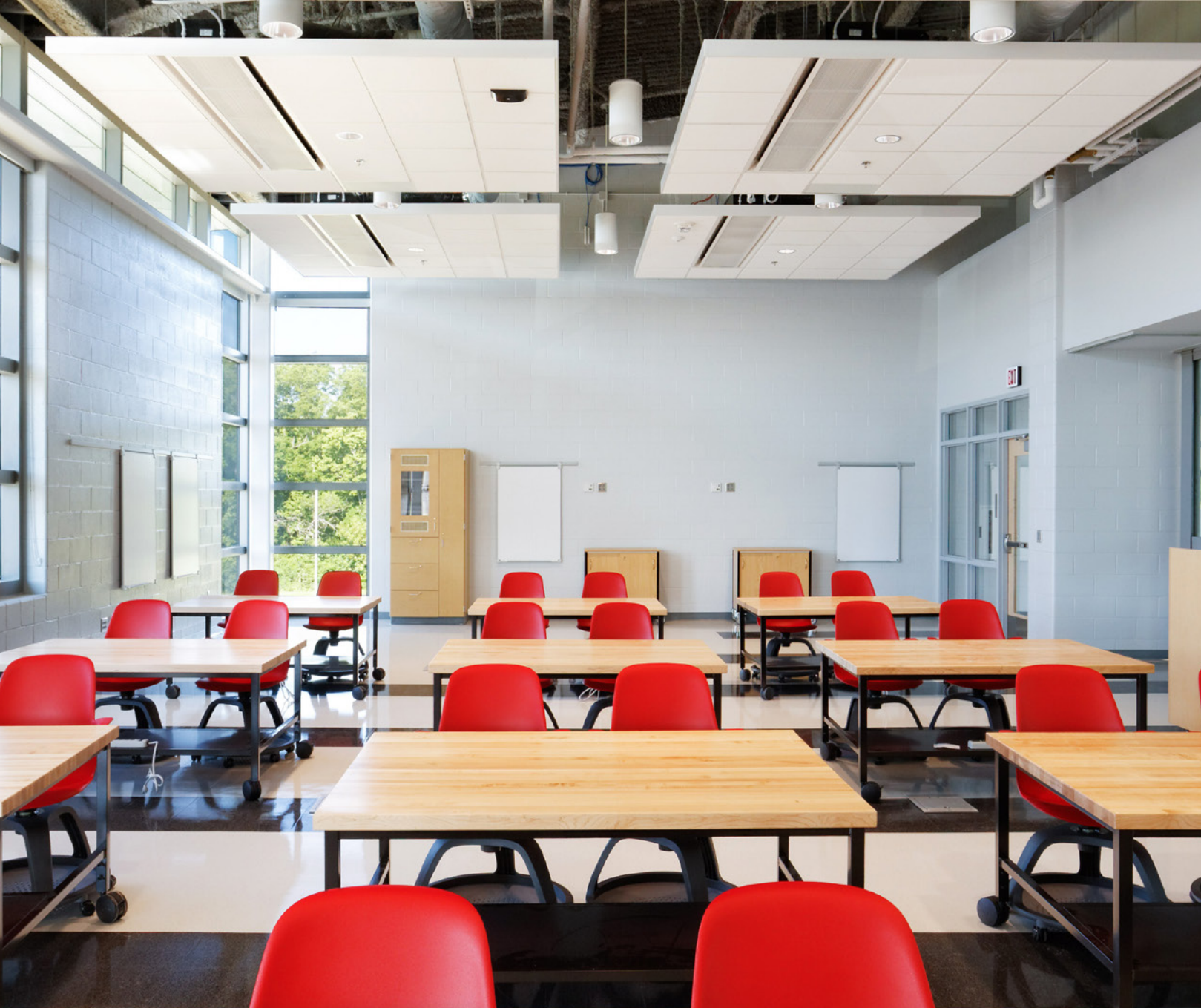
Classroom Layout: Overhead Mixing with Chilled Beams
