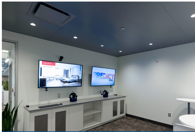
SQUARE PLAQUE DIFFUSER (SPD) in Armstrong Torsion Spring Ceiling with Coordinated Finishes
